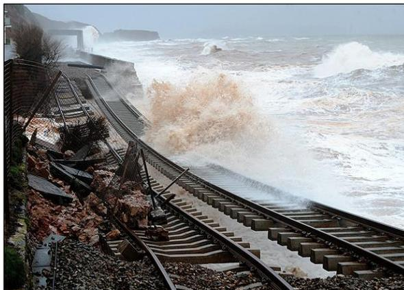
**Figure 1: Dawlish rail line damaged due to 2014 coastal storms, Devon, UK.<sup>234</sup>**
